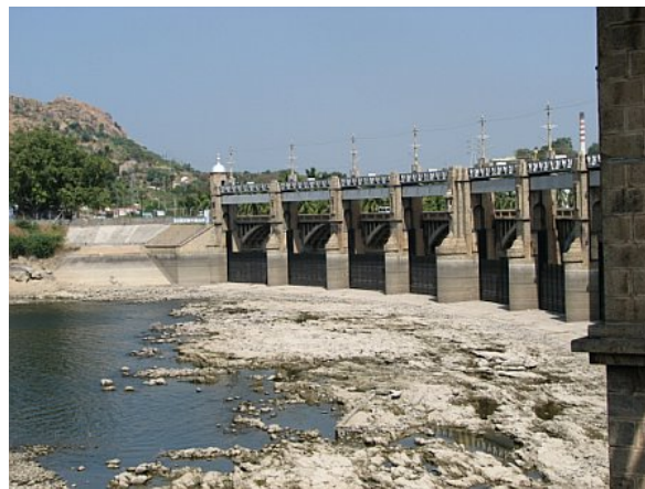
Mettur Dam crest gates
